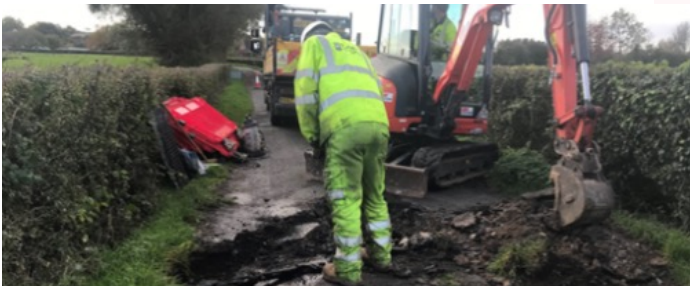
Repairs being undertaken along Badger Lane , Pawlett
