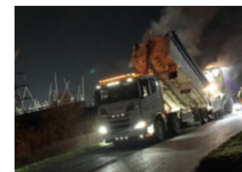
Nightworks on the C182 (access road to Hinkley Point C)
