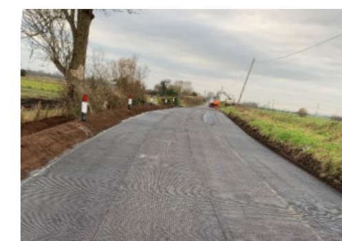
Use of geotextile at Meare Road, Glastonbury
