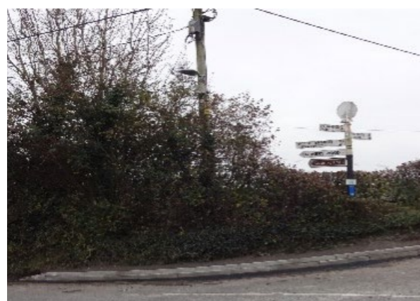
Junction improvements at Rudge Lane, Beckington
