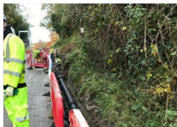
Drainage improvements at Winsford
