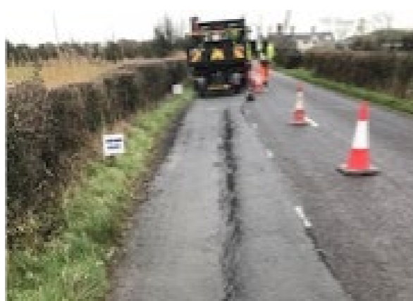
Edge Repairs at Lympsham
