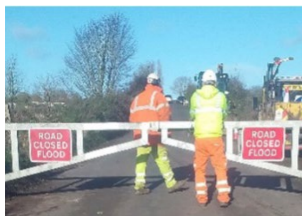
Refurbishing Lyng Floodgate
